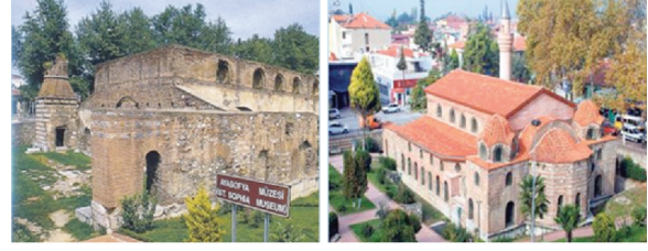
Figure 6. Before and after restoration of Hagia Sophia Museum [11]
